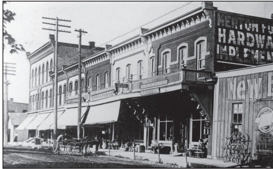
The Cooper Block is still standing along Richmond's Main Street south of Monroe.
