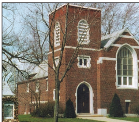
St. Andrews Church after removal of the ivy
