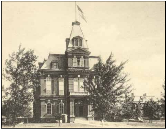
Sandusky courthouse built in 1879 burned down 1915 was built by Arthur Carson, who is believed to be one of Sandusky’s first settlers. Even when road construction began, the conditions were See SANDUSKY, Page 18
