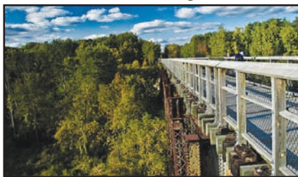
The old railroad bridge on the Wadhams to Avoca Trail.
