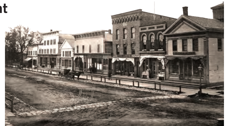
The west side of South Main Street circa 1894
