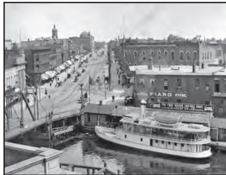
Port Huron circa 1910, Huron Street and ferry landing
