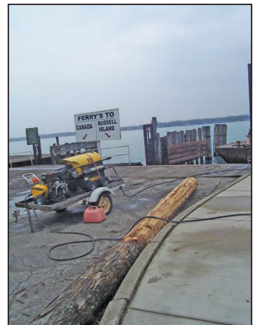
The replacement for the broken pylon
