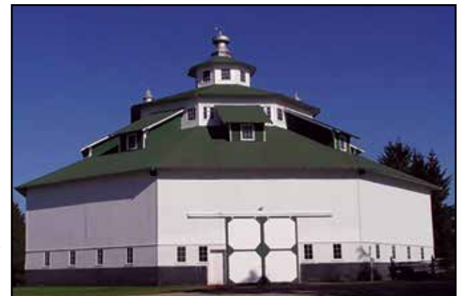
The Thumb Octagon Barn and Agricultural Museum is located at 6948 Richie Rd in Gagetown, Michigan.
