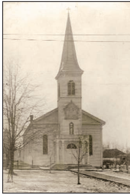
The former Immaculate Conception Church was destroyed by fire in 1917.
