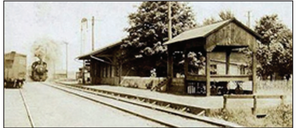
Train traveling south, from Port Huron, into the New Haven Depot
