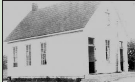
Harris School on New Haven Road near Place Road
