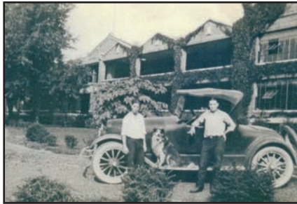
The former St. Clair County Infirmiry and Medical Center was demolished in 1992.
